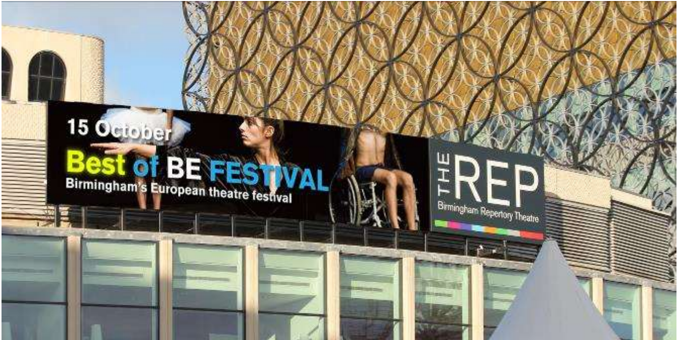
Above: Full colour video board, 11.2 x 2.5 metres. Video, animation and text can be used to stunning effect to promote the upcoming events at the venue. Birmingham Rep Theatre
