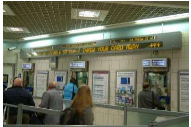
Above: Liverpool Street Station ticket kiosk main display comprising 56 character 140mm main message display with 3, 60mm 16 character call forward displays above each booth. A button activated call forward PA system also included.
