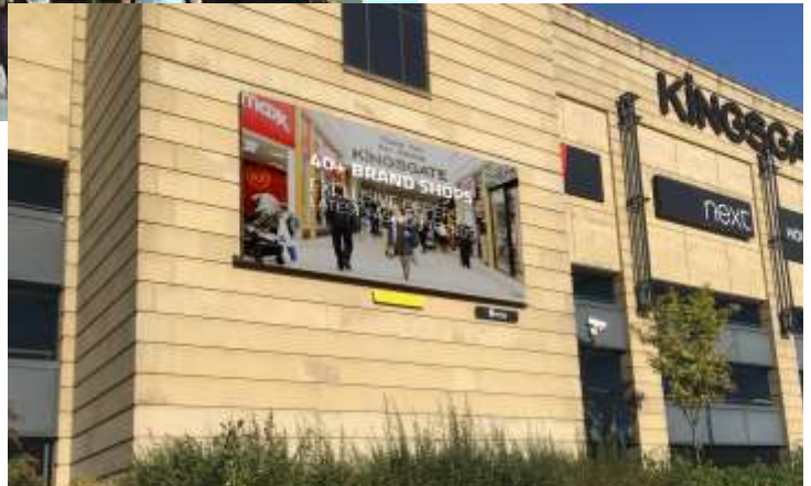
Right: Full colour LED video display, Installed as you enter the shopping centre.
