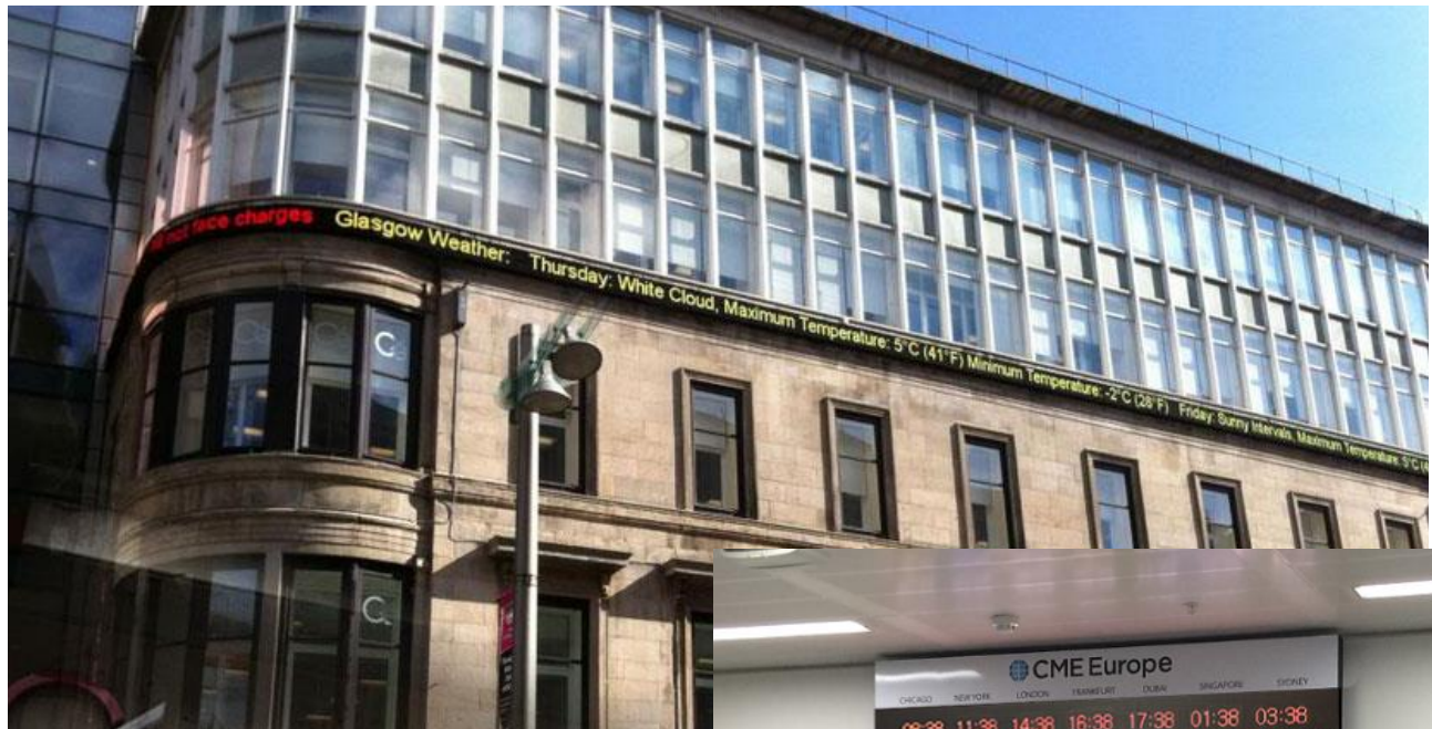
Above: External curved full colour LED ticker installed at the Clydesdale bank. Although the display can show various text heights and graphics, it is shown here running 350mm high text
