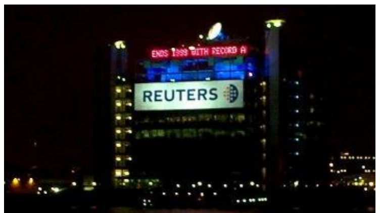
And Below: At the turn of the Millennium we installed this 42 metre long Ticker display on the roof of the Reuters building in London. It was the biggest outdoor display at that time. Making history again!
